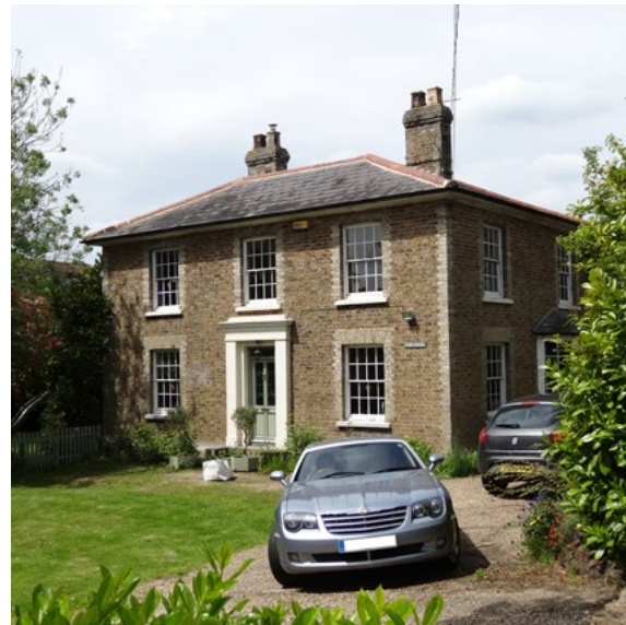
Fig 1.72 - York House, Kelvedon Road.
