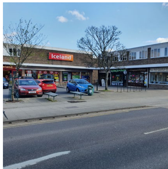
Fig 1.53 - Shops along Church Road
